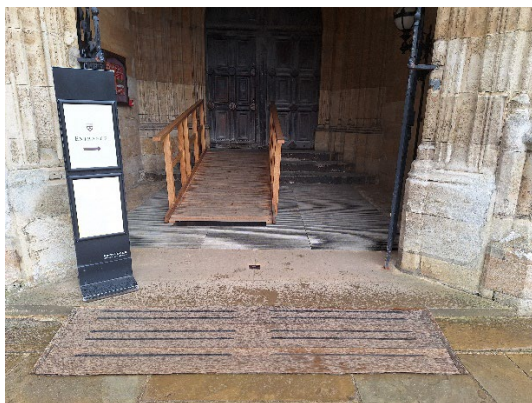
Ramped entrance (South Door – main entrance)
